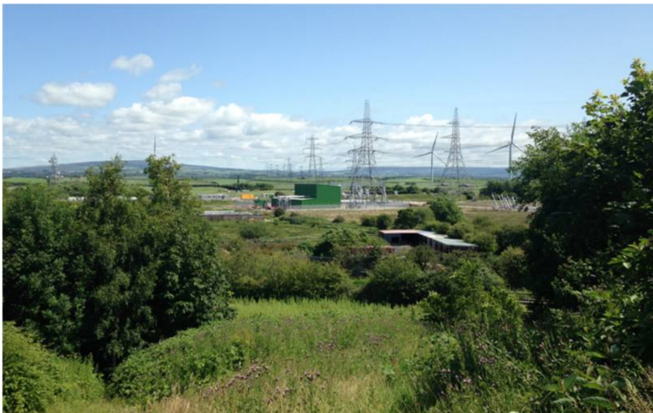
Image 3.5 Existing Middleton 400 kV Substation (Source: National Grid)
